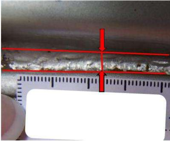
Visible blisters have spread more than 5mm from inner edge of paint sealer
