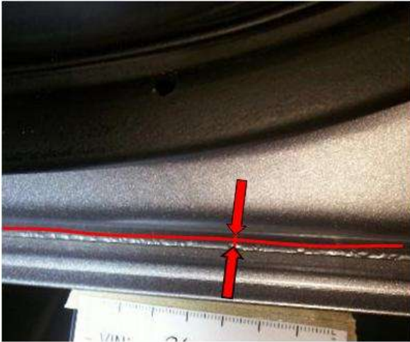
Maximum width of blisters is less than or equal to 5mm from inner edge of paint sealer.
