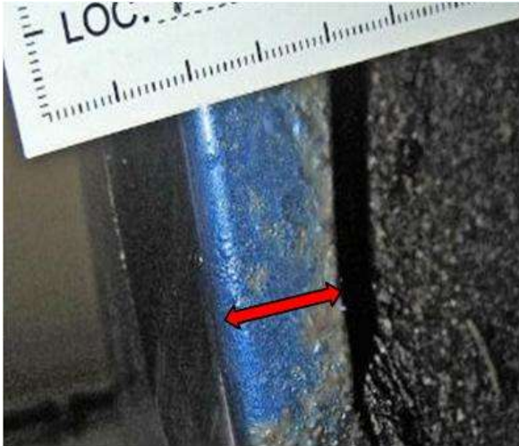
Visible blisters and red rust in an area more than 10mm from the inner edge of the wheel arch.
