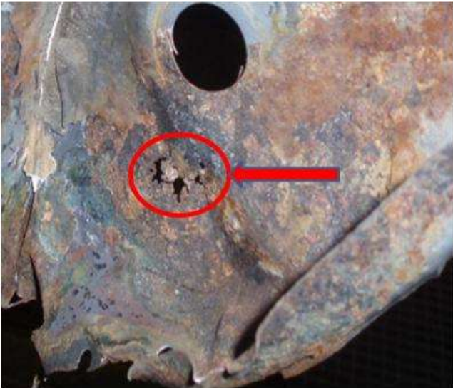
Part of the inner wheel house is perforated by corrosion from the outside.
