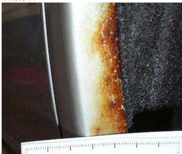
Red rust in an area more than 10mm from the inner edge of the wheel arch.
