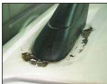
After rain, acidic water gathered partially, penetrated in the paint and caused peel-off. ( roof rail )
