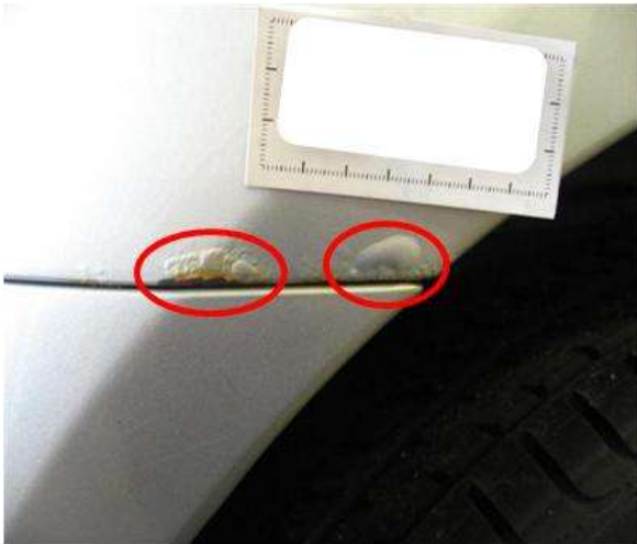
Visible blisters and red rust at vertical surfaces of wheel arch or rear bumper attachment area will not lead to level-3 as long as no proof for perforation can be detected.
